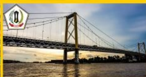
Jembatan Barito, Kab. Barito Kuala
