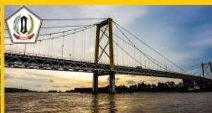
Jembatan Barito, Kab. Barito Kuala
