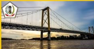
Jembatan Barito, Kab. Barito Kuala
