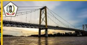
Jembatan Barito, Kab. Barito Kuala
