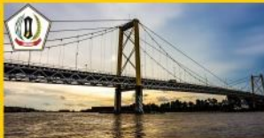
Jembatan Barito, Kab. Barito Kuala
