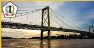
Jembatan Barito, Kab. Barito Kuala
