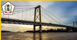
Jembatan Barito, Kab. Barito Kuala
